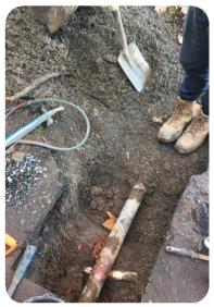
When permitted, potholing needs to be undertaken with extreme care and by employing techniques least likely to damage assets. Remember if machinery is on site it can come into contact with overhead power. Refer to 'look up and live' on the following page.
